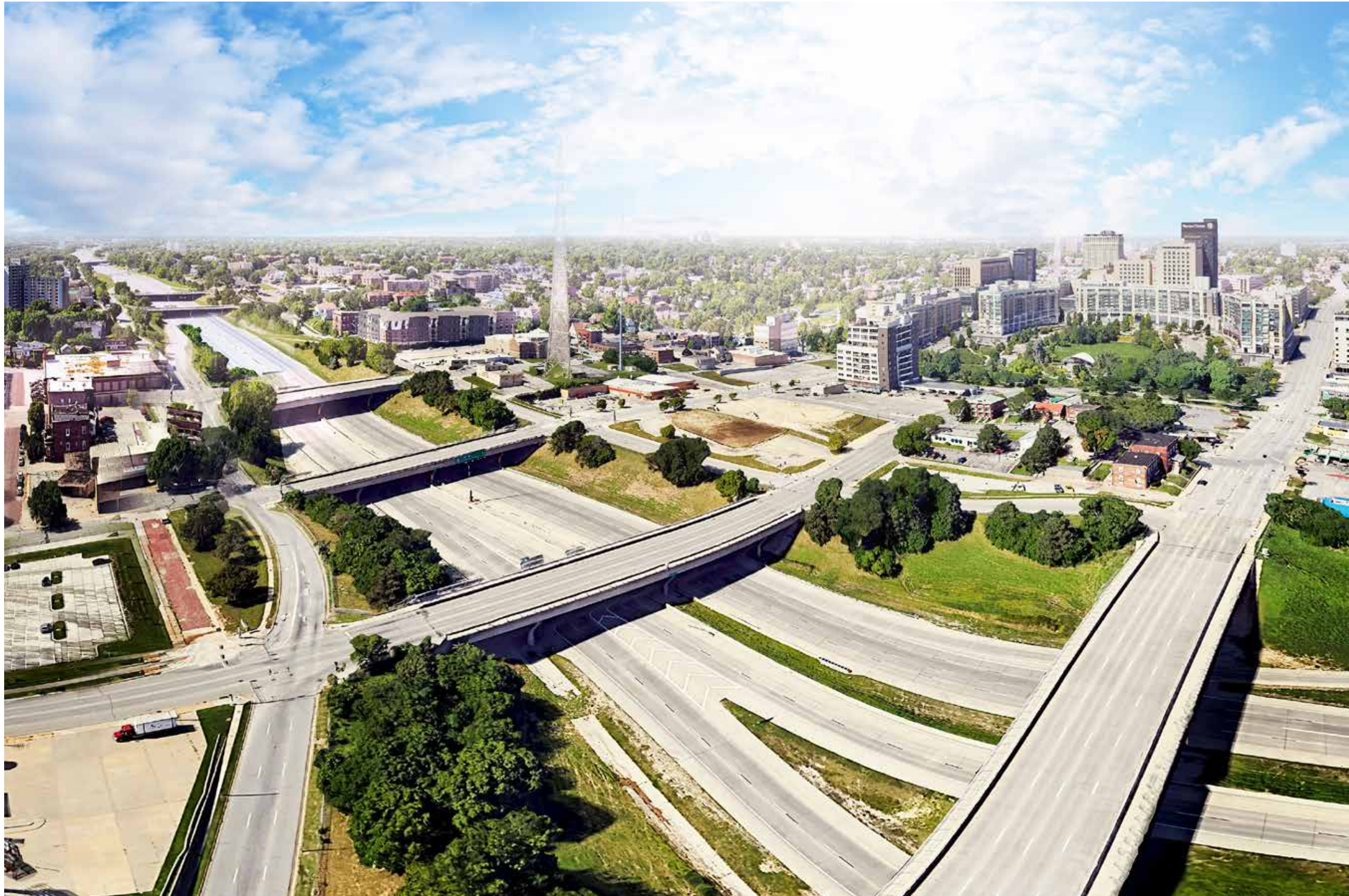
Left: BEFORE Photo of existing conditions looking to the southwest towards Midtown Crossing, showing the Harney, Farnam, Douglas, and Dodge street bridges over I-480.
