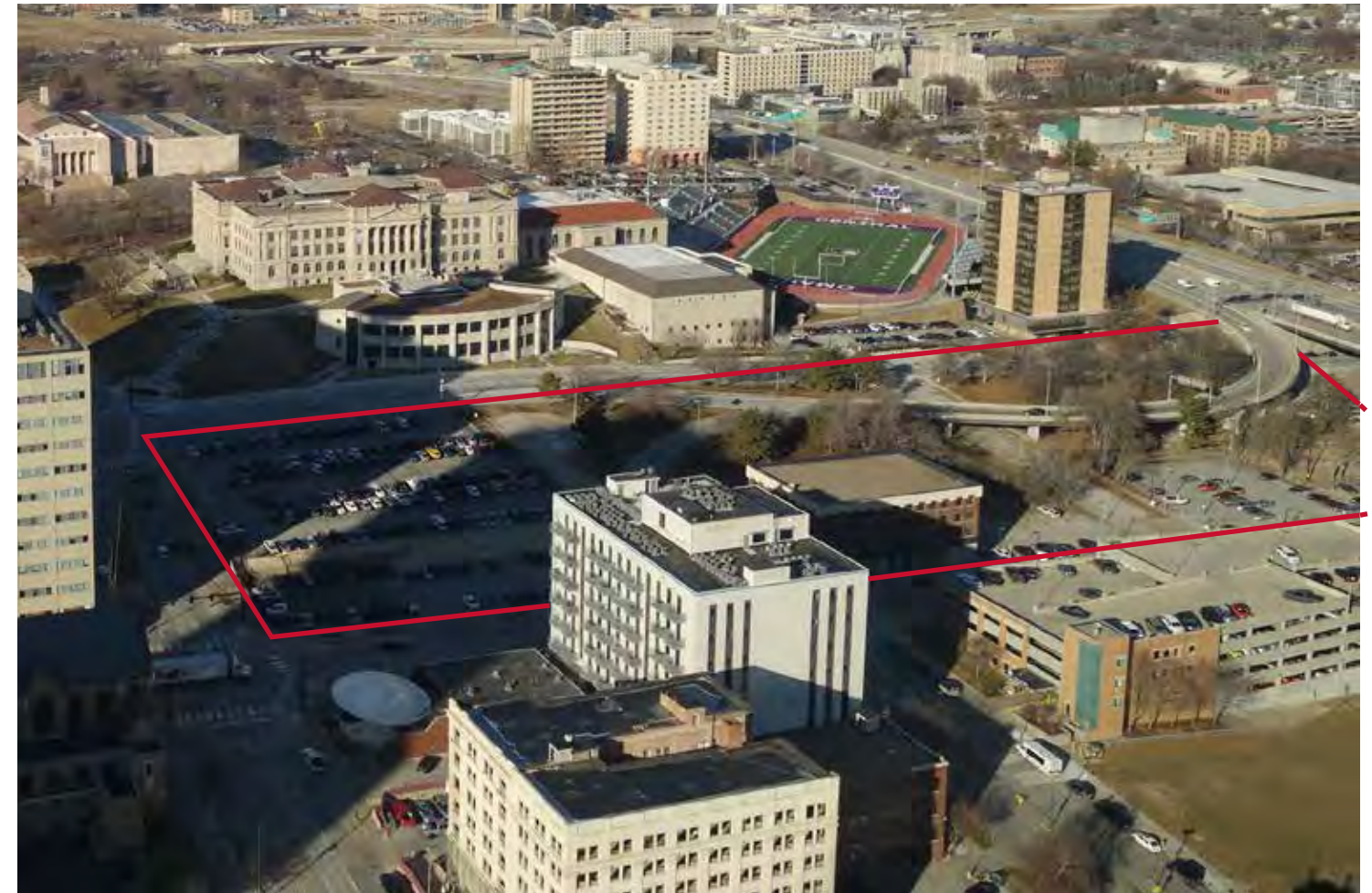
Aerial photo of existing 19th & 20th Street Ramps
