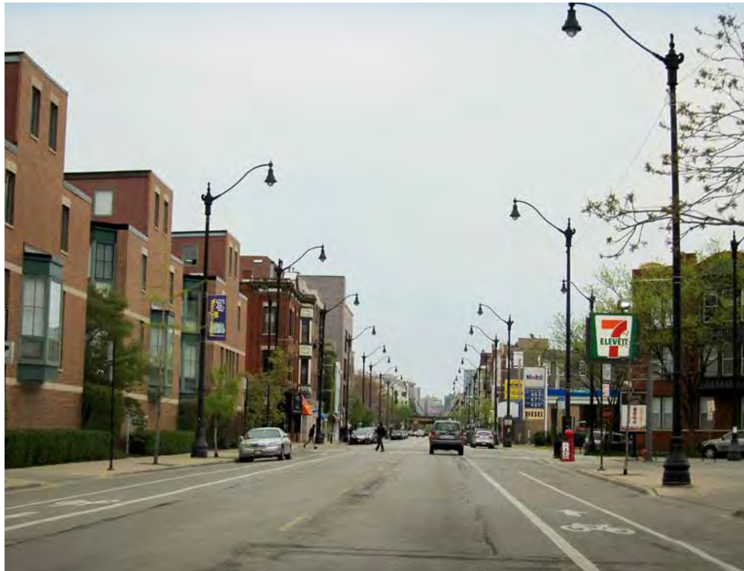
Example of a "B" Street
