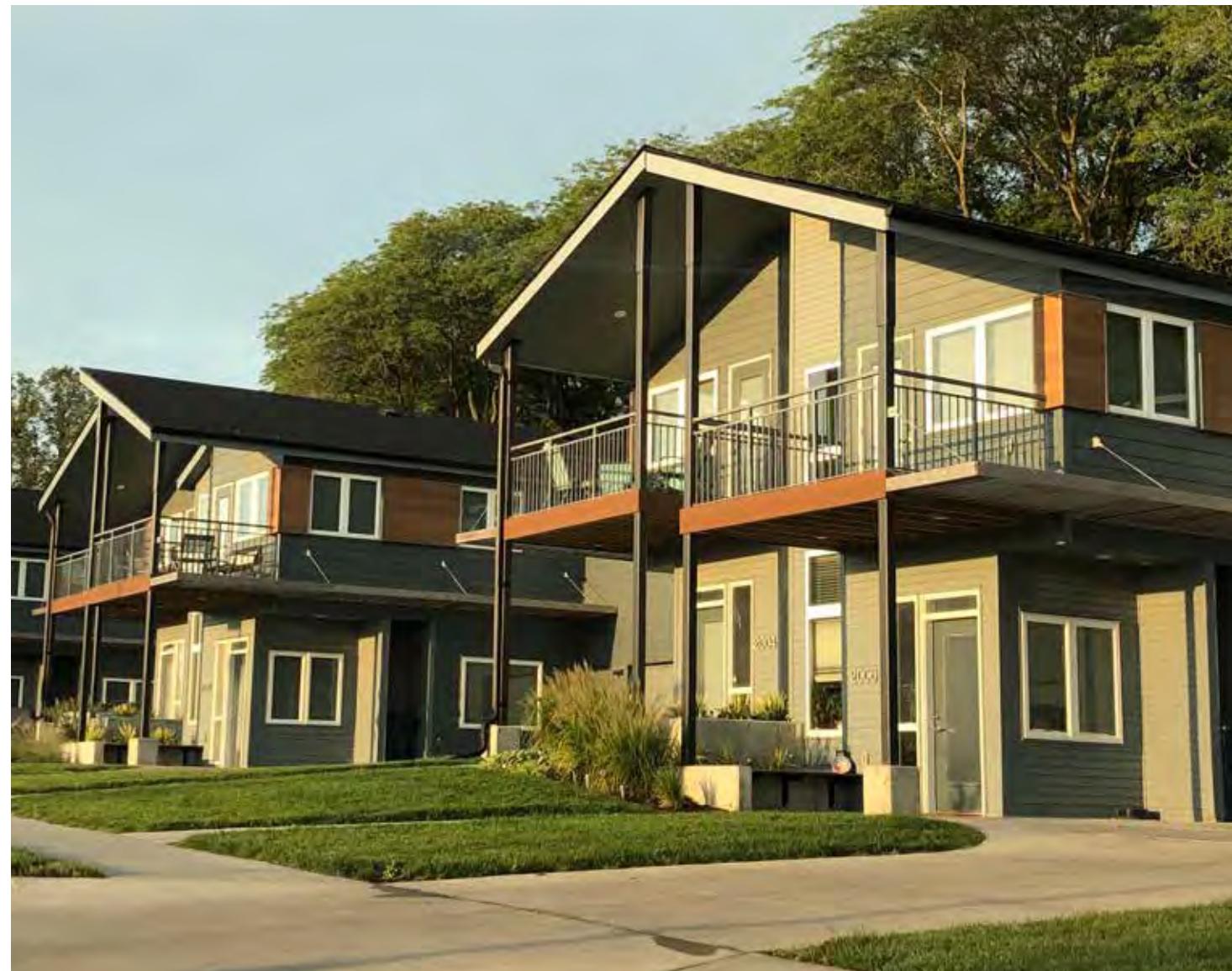
Housing within Reach at 75 North
