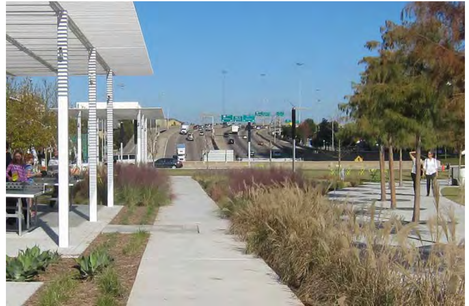
Klyde Warren Park, a LID over the Woodall Rogers Freeway in Dallas, TX
